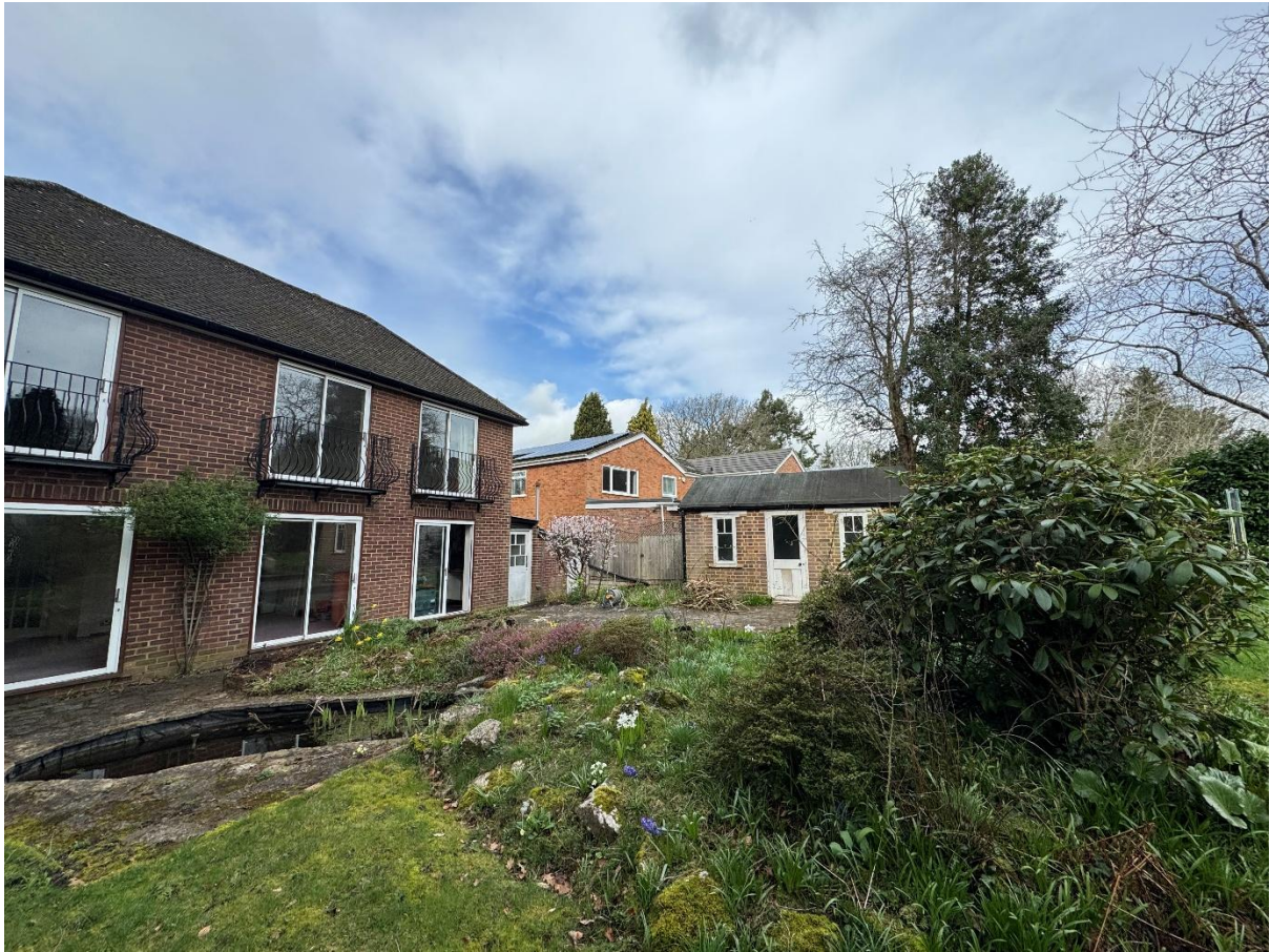
Figure 2: View of No. 18A
