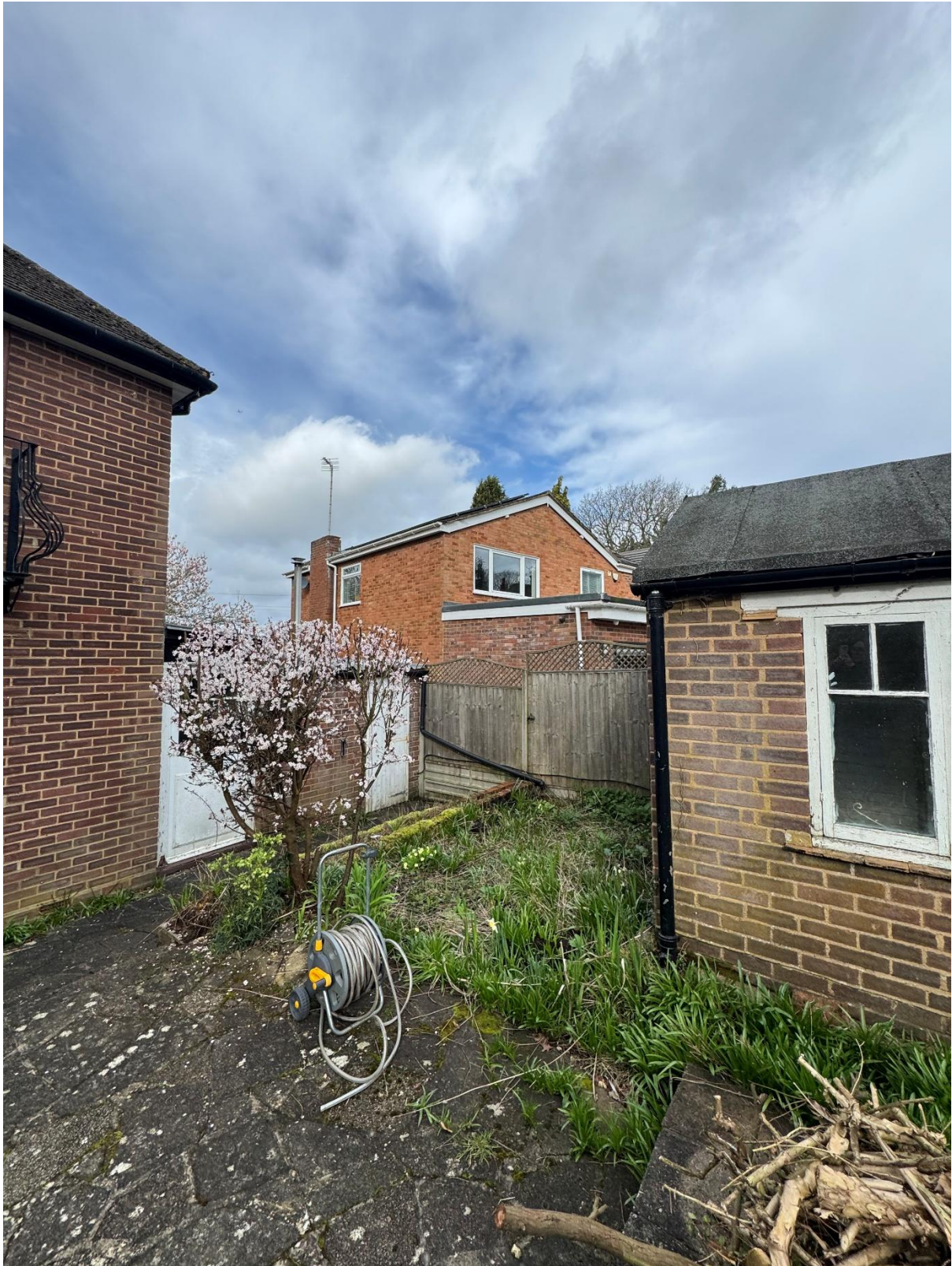
Figure 6: View towards 18A
